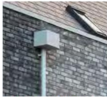
Rectangular metal rainwater pipe and hopper powder coated. Colour: TBA to match with window frames and balcony metal railings
