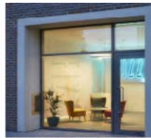
Communal entrance door - Factory colour-coated proprietary curtain walling system with glazed entrance door with GRC surround
